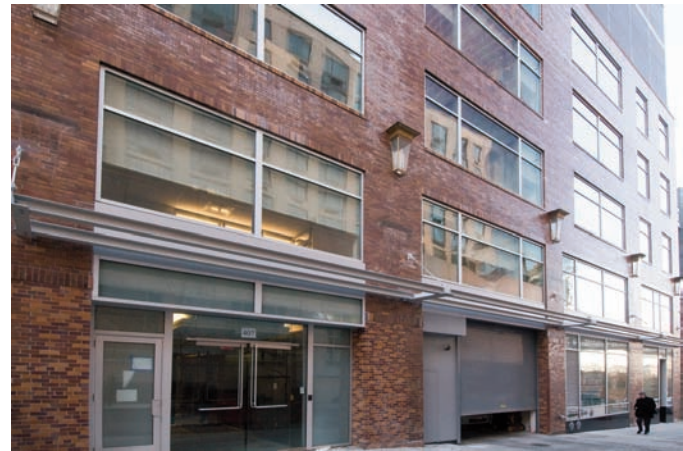
Once a Rolls Royce showroom and the a parking garage, 407 East 61st Street is now a beautiful addition to the street and provides state-of-the-art space for research labs and administrative offices.
